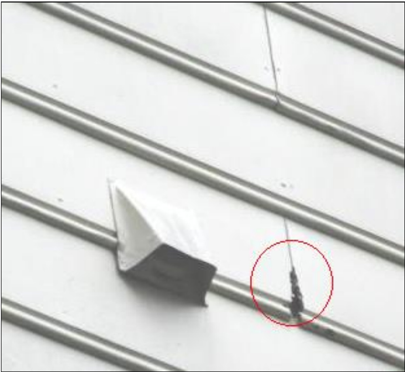
1.9 Item 8(Picture) Damaged End Joint Left Side
