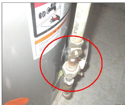
9.6 Item 2(Picture) Original Gas Shut Off
