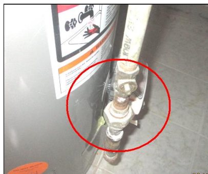
9.6 Item 2(Picture) Original Gas Shut Off
