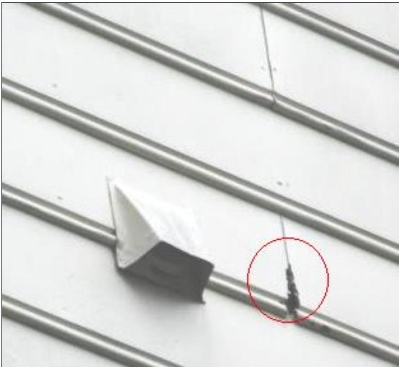
1.9 Item 8(Picture) Damaged End Joint Left Side
